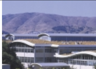
GAP Headquarters San Francisco, CA William McDonough and Partners, Architects Uses AAC SolarTrac System
